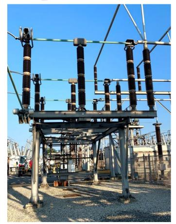
*Figure 1*: 345 kV Disconnect Switch w/Center-Pivot Horizontal Swing Arms [1]
